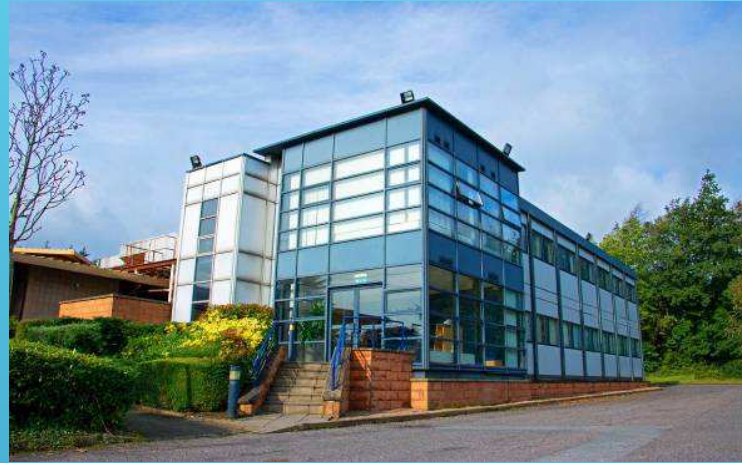
Northern Ireland factory
